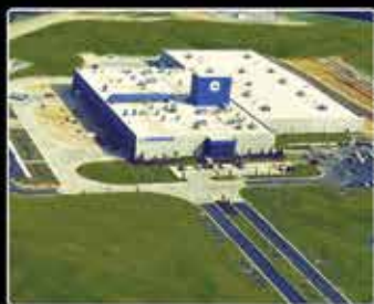
PAGELAND, SC Bronze Foundry and Manufacturing Plant
