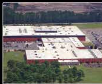
CONWAY, SC Steel Foundry and Manufacturing Plant
